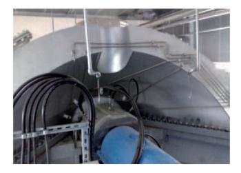
Risks: The fire hazard emanates from flammable liquids that spread over hot surfaces due to leaks in the lubrication or control oil system.
