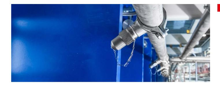
A distinct fire risk can also be identified in the pit below the press – e.g. from hydraulic or thermal transfer oil equipment and accumulated fibers and grease. This particular risk should be protected as a separate extinguishing zone with the addition of a special foaming agent.
