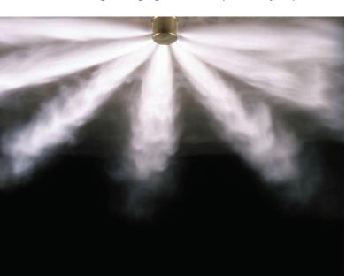
Therefore, HFC-227ea is neither corrosive nor electrically conductive, leaves no residue and can easily be removed from the space concerned through ventilation. HFC-227ea is, besides inert gases, the preferred extinguishing agent for electronic and electrical risks.
